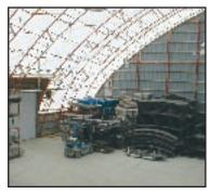
The 90' to 160' wide series of **Diamond Shelters** have welded truss end frame poles. Such a design is necessary to withstand higher wind loads.
