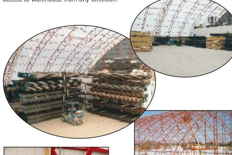
All Diamond Shelter frames are constructed of hollow structural tube with yield and tensile strengths that allow them to withstand heavier stress loads. All frames are engineered to meet requirements of the National Building Code.
