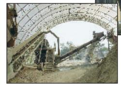
All rafters and cross bracing have easy to assemble, bolt together joints.
